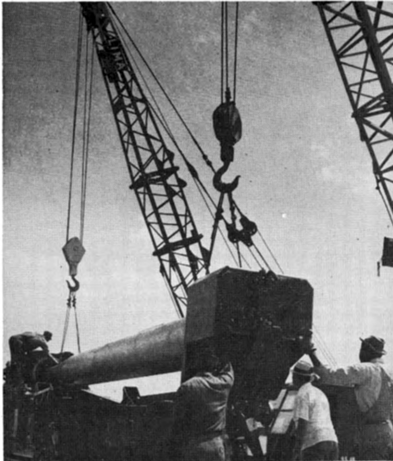
A CLOSE FIT . . . Atomic needle threading by two mobile cranes completed an almost impossible job of inserting the firing tube into the carriage of the 280 mm cannon from two separate railroad cars. Due to lack of special equipment, Infantry Center personnel had to improvise this system of putting the gun together.
